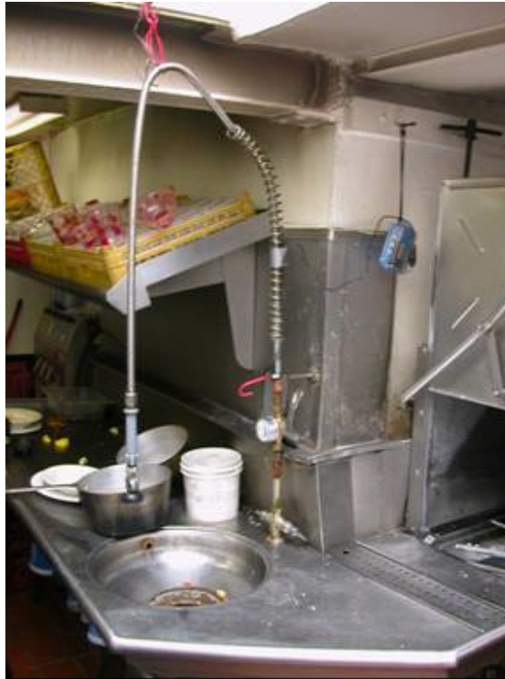
Figure 13. Meter Installation Showing Data Logger Case
