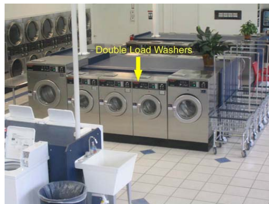
Figure 13-8 Double-load machines ( > 20 pounds clothing)
