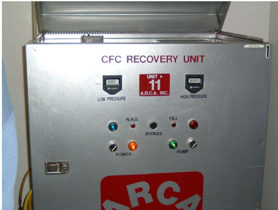
Figure B-6 CFC-11 Recovery Equipment
