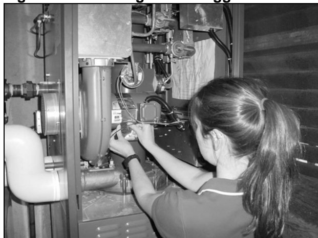
Figure 3.3 Installing Motor Logger
