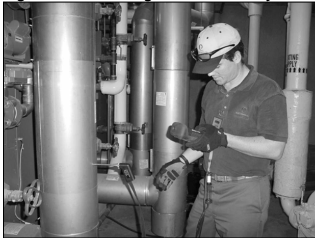
Figure 3.1 Measuring Boiler Efficiency
