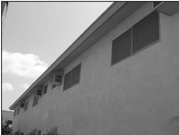
Fig. 3.3 Flanders Pointe Solar Sunscreens
