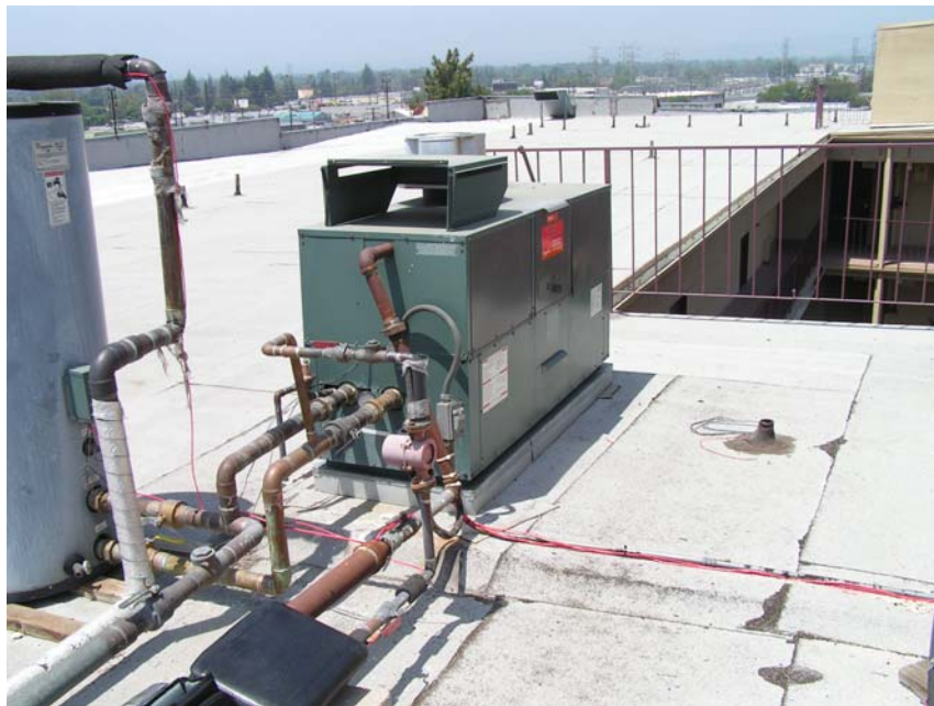
Figure 5 Unprotected Control Connections
