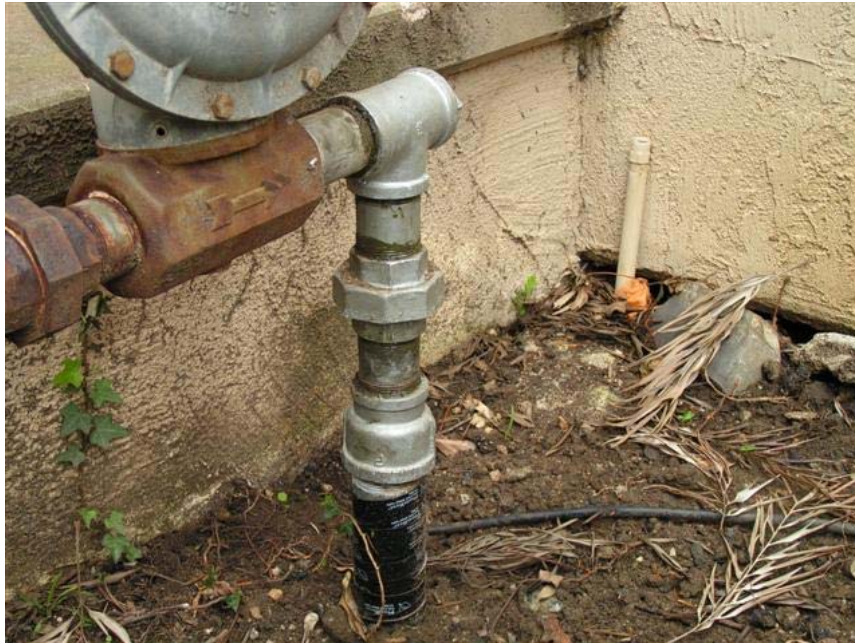
Figure 8 Replaced Gas Piping
