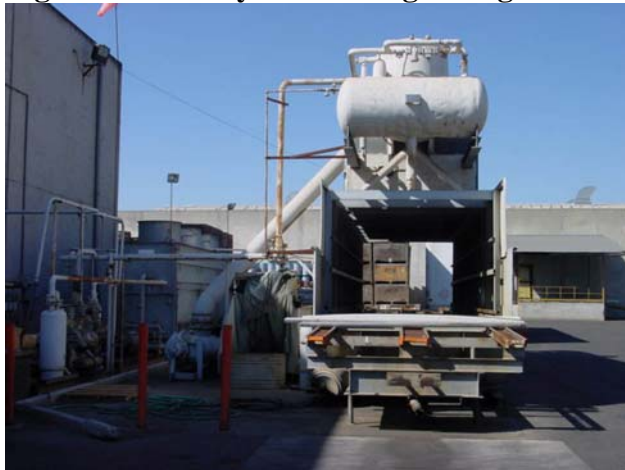
Figure 5.2 Old Hydro-Cooling Refrigeration
