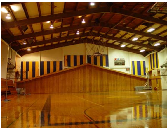
Figure 1. Pre-Retrofit HID/Incand. Fixtures
