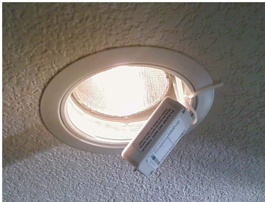
Figure E-6: LL Logger Installation in a Downlight w/ Zip ties
