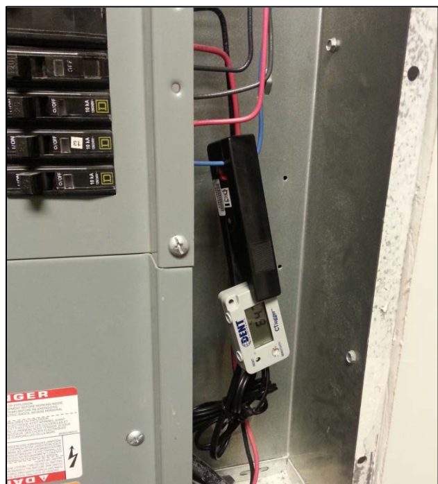
Figure E-4: Dent CT Logger on Circuit in Electric Panel
