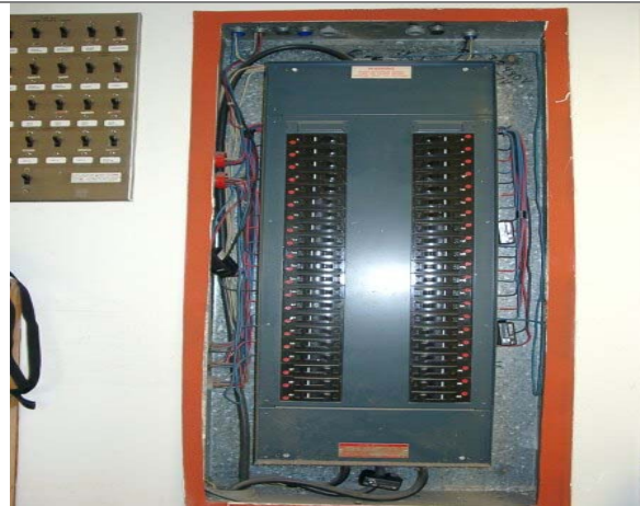
Panel A With Dataloggers
