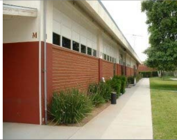
Building M Outside
