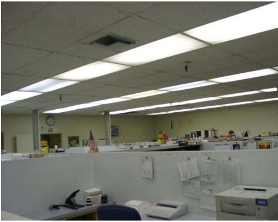
Front Office, Bullpen Fluorescent Lights
