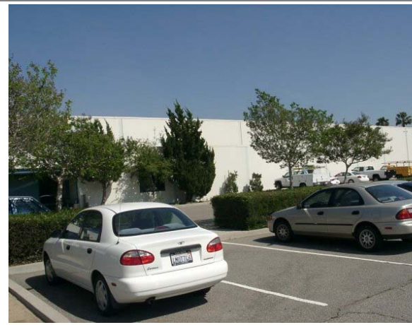
Castaic North Services Building Front
