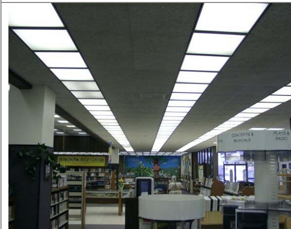
4-lamp 4-Foot Fluorescent Fixture Rows
