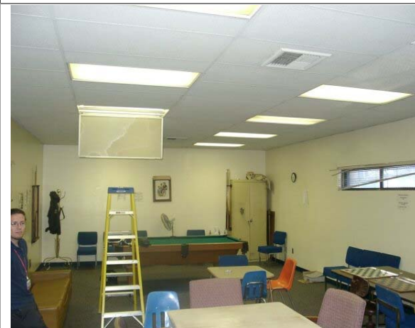
Game Room T-12 Lighting Fixtures
