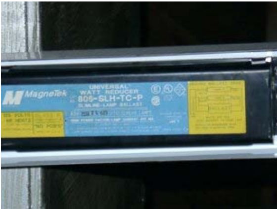
Warehouse 8' 2-lamp Ballast
