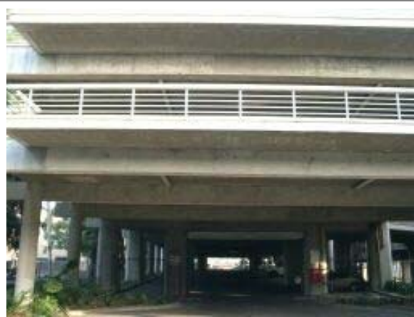
Bellflower Parking Structure
