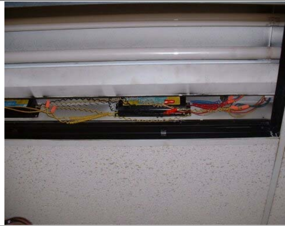
Old T12 Recessed 4-Lamp Fixture
