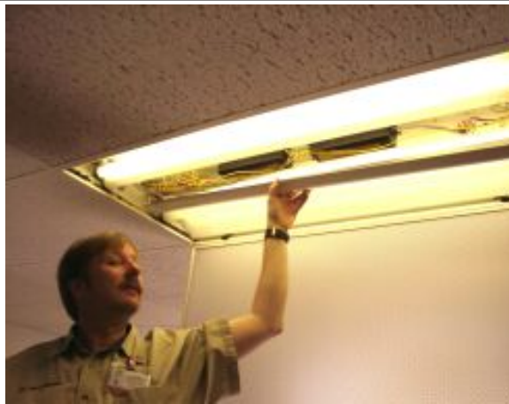
Dr. Mark Shirilau, Inspecting a Lighting Fixture
