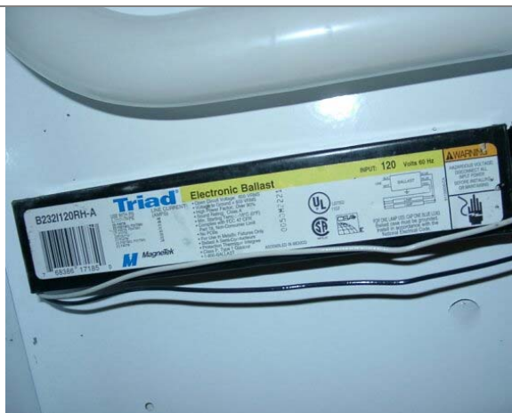
Kitchen U-Bend Fixture Electronic Ballast
