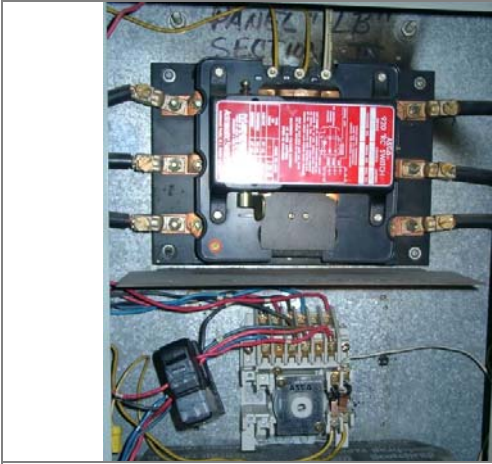
Contact Timer With Datalogger (Top)
