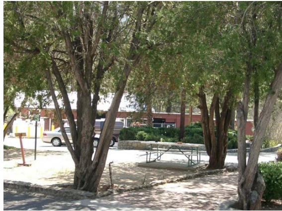
Maintenance Shop Building
