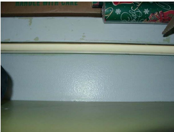
Hidden Fixtures In Observation Room
