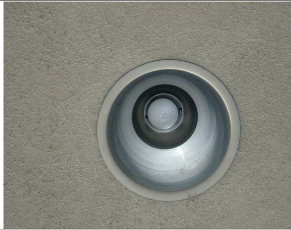
Exterior Recessed HID Fixture
