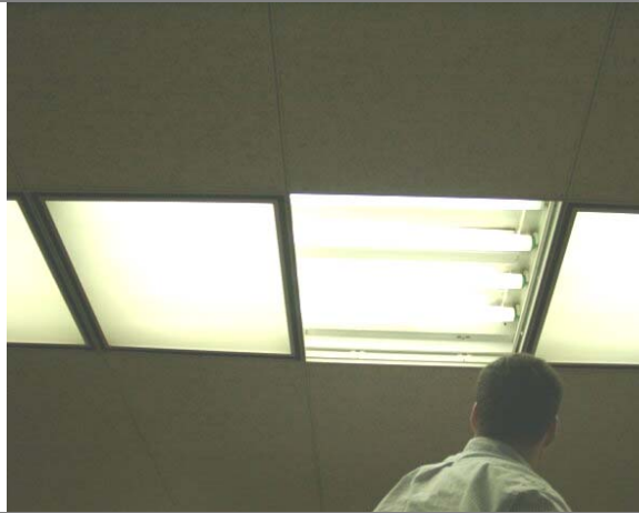
4-lamp 4-Foot Fluorescent Fixture Row
