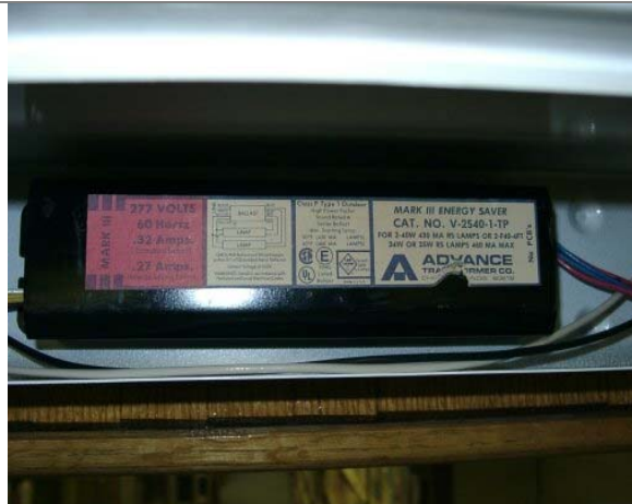
1x4 Wall Mounted Strip Ballast
