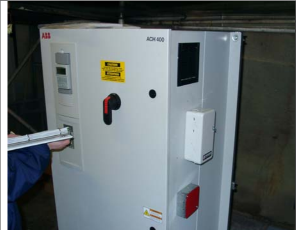
W-81 Room New VFD System with Timer
