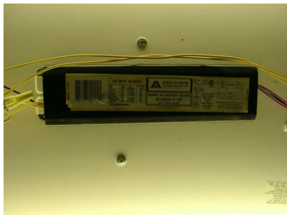
2-lamp Energy Saver Magnetic Ballast
