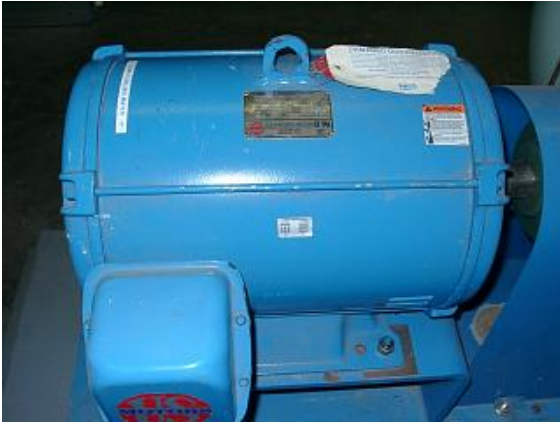
New Chiller 25hp Motor
