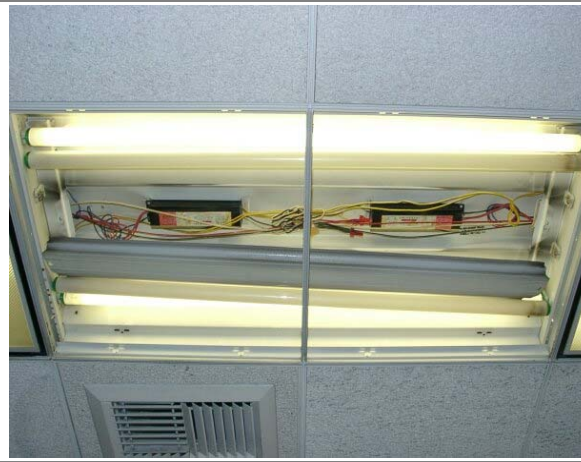
4-lamp 4-Foot Fluorescent Fixture Ballasts
