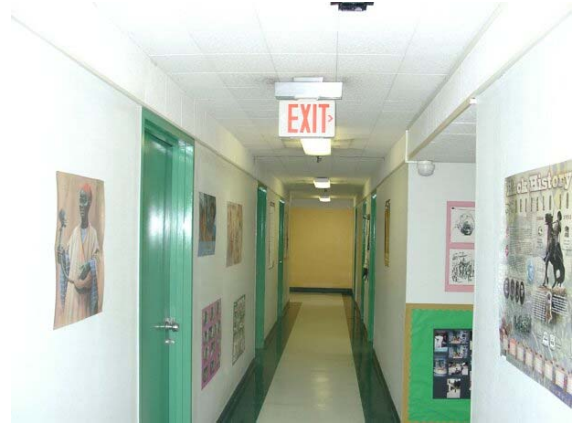
Hallway Fixtures And Exit Sign
