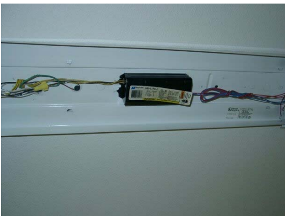
Wrap Fixture Ballast in Warehouse Office
