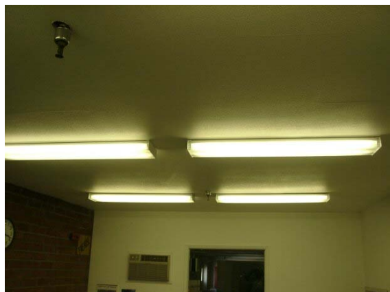
Wrap Fixtures in Office Area
