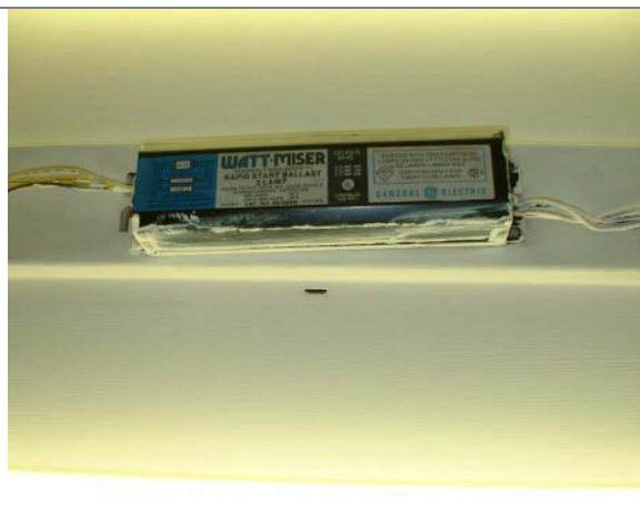
Rapid Start T12 Energy Saving Ballast
