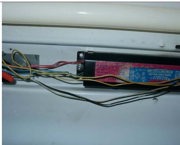
2x2 Fixture Ballast
