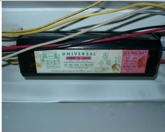
A 2-lamp 277-volt Fluorescent Ballast
