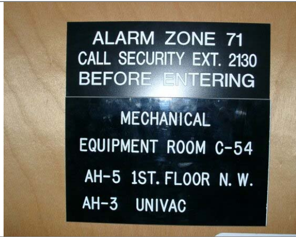
C-54, Downstairs West Air Handler Room
