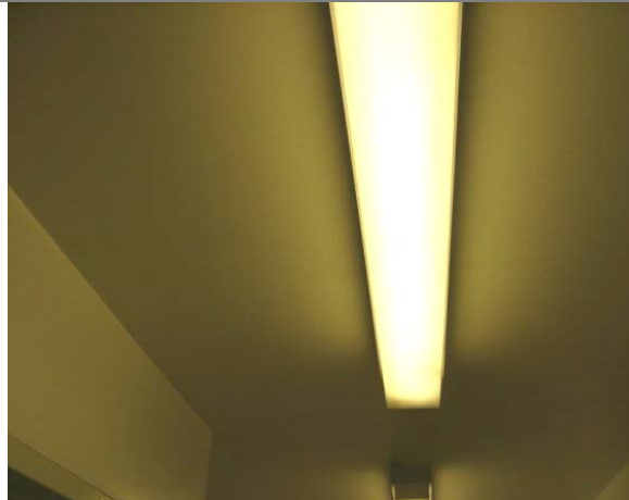
Restroom 2-lamp Surface Mount Fixture
