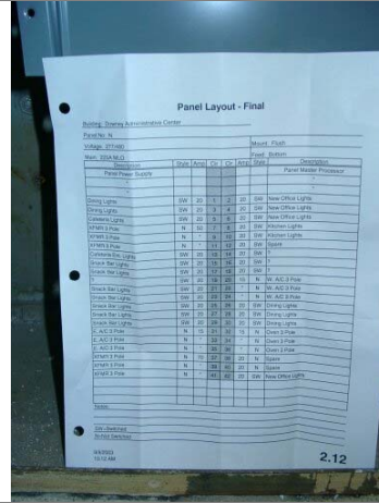
New Lighting Breaker Panel N Legend
