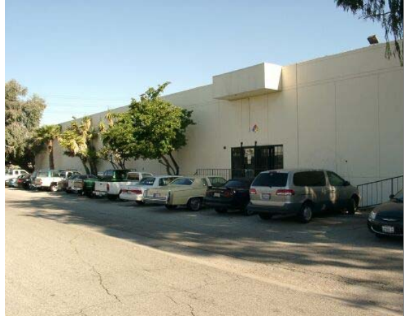
ISD - Dist. 3 Facilities Building
