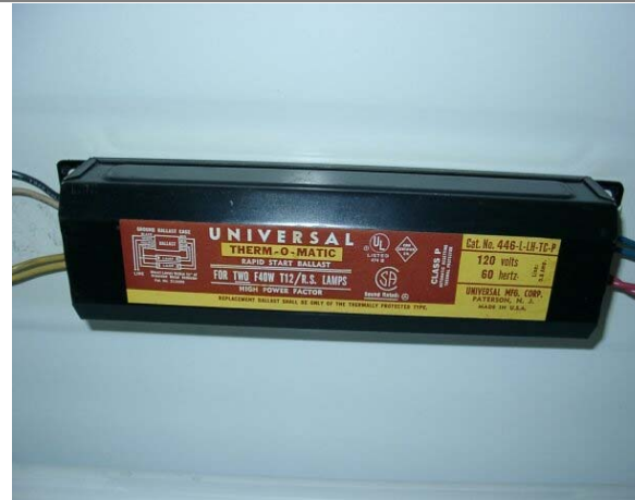
Office Hallway 2-lamp Fixture ES Ballast
