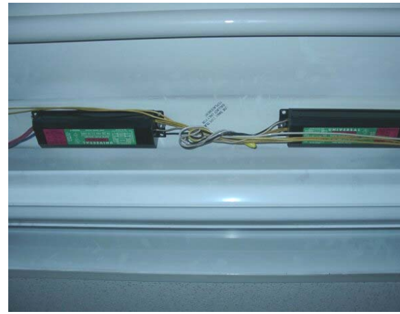
4-lamp Office Light Fixture, ES Ballasts
