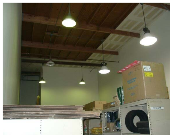
Warehouse Storage Area HID Fixtures
