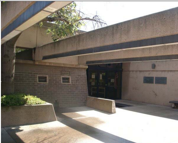
Claremont Library Main Entrance
