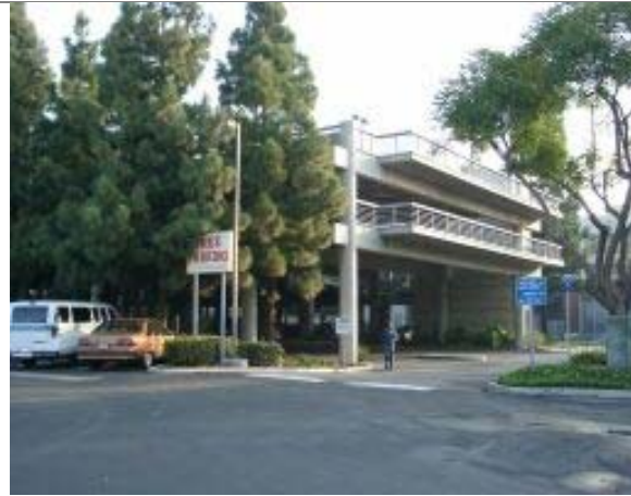
Bellflower Parking Structure
