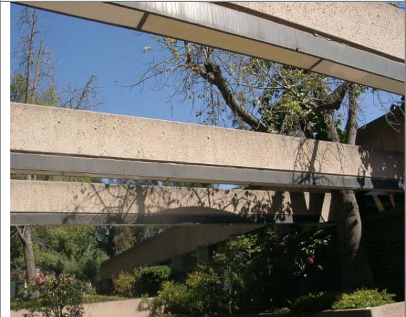
Outdoor 1 x 4 Strip Fixtures, By Entrances
