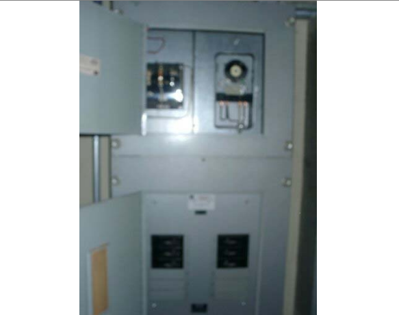
Parking Garage Panels
