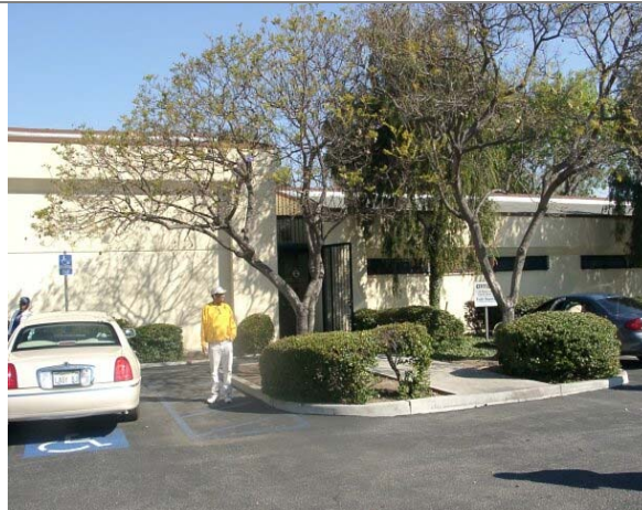
Willowbrook Senior Center Building
