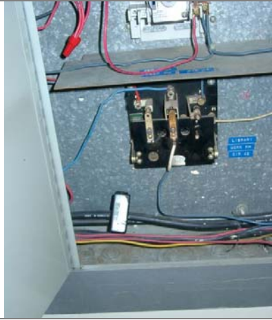
Contactor With Datalogger (Bottom)
