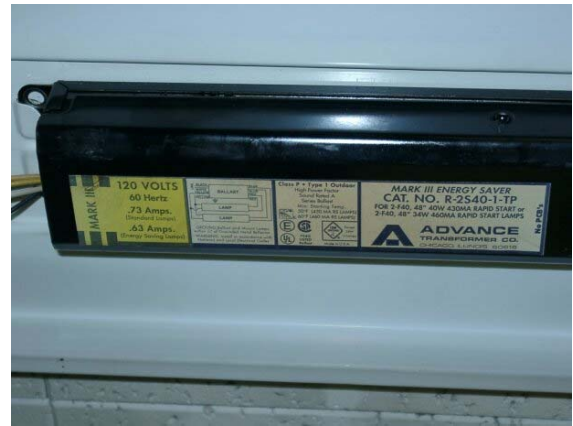
Surface Mounted 2-lamp Fixture Energy Saver Ballast
