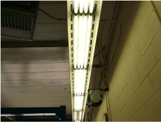
Auto Shop Lighting 4-lamp Old Light Fixtures
