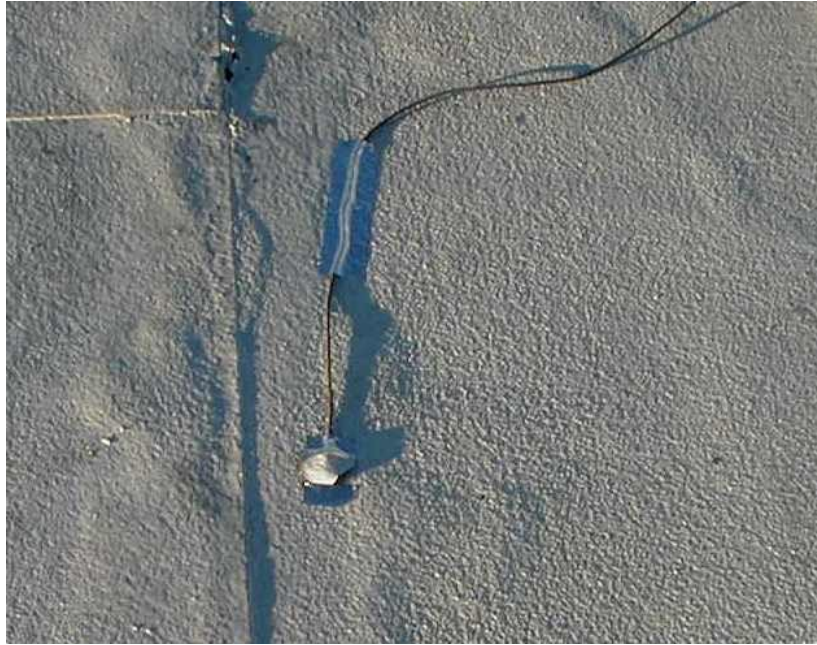
Figure 5. Coated Store Roof Temperature Sensor
