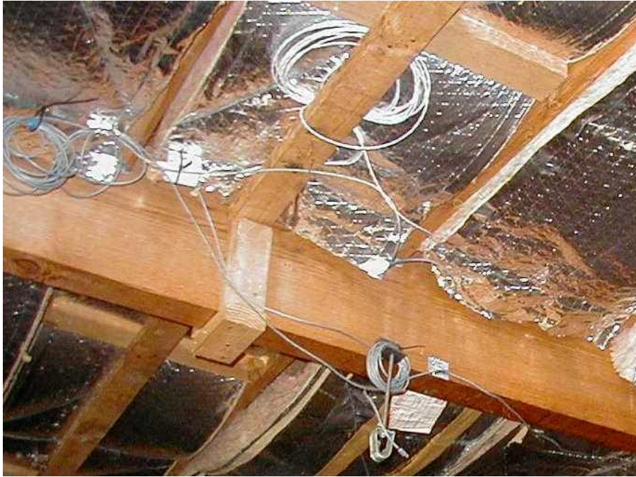
Figure 7. Deck Logger Installation
