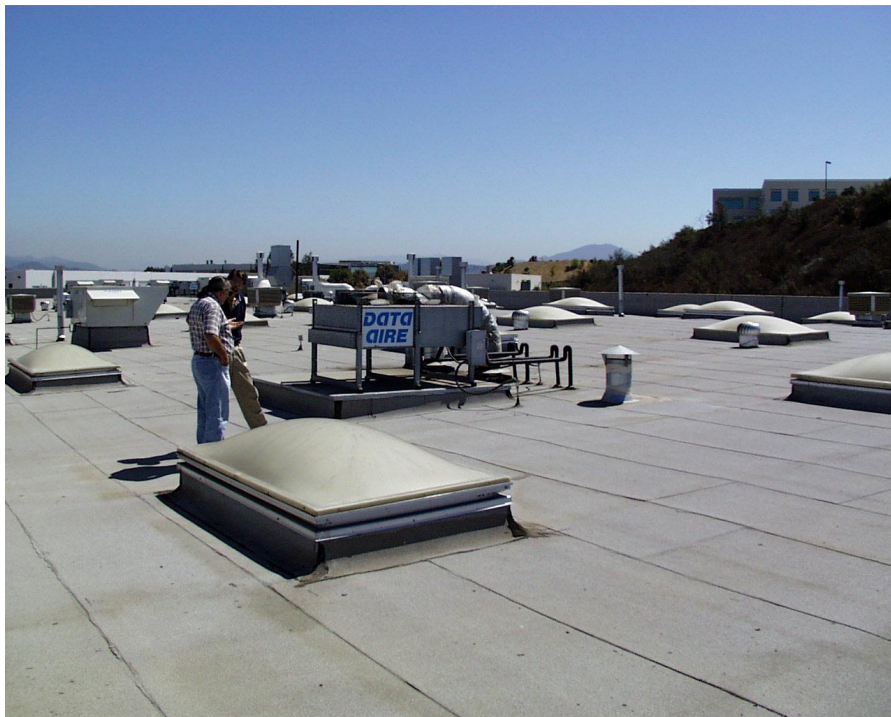
Figure 2. Site A Roof
