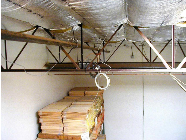
Figure 5. Deck Logger Installation
