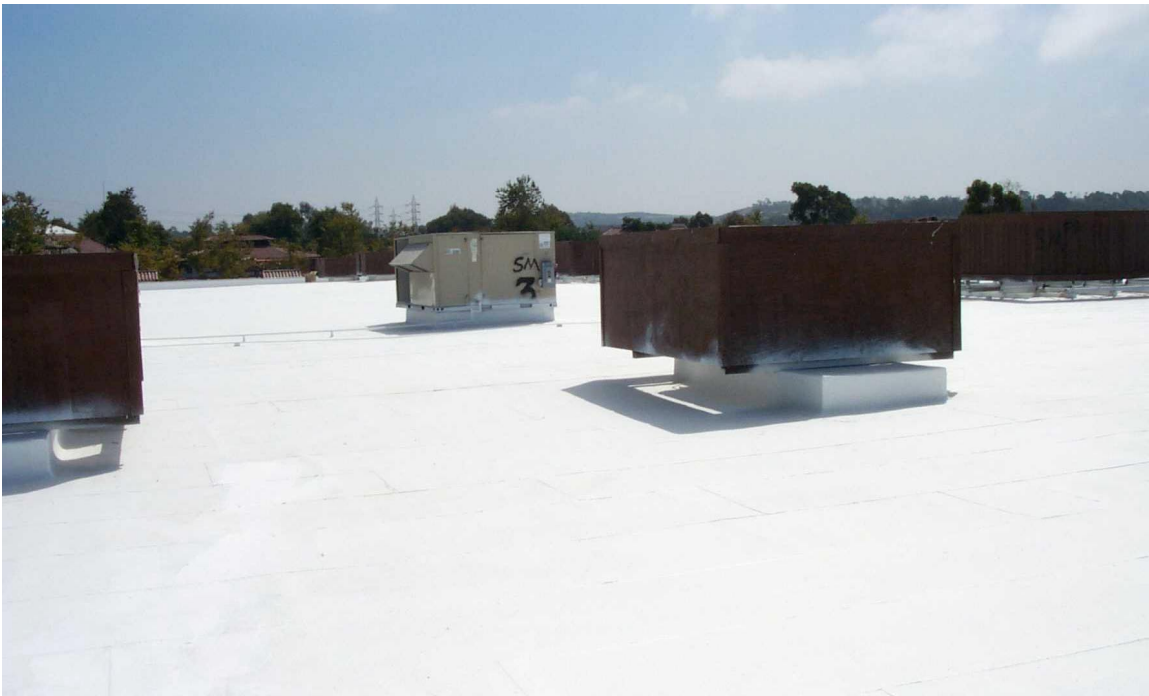
Figure 3. Coated Store Roof
