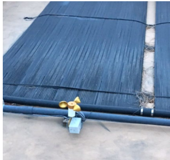
FIGURE 2-12: EXAMPLE OF ANEMOMETER INSTALLATION
