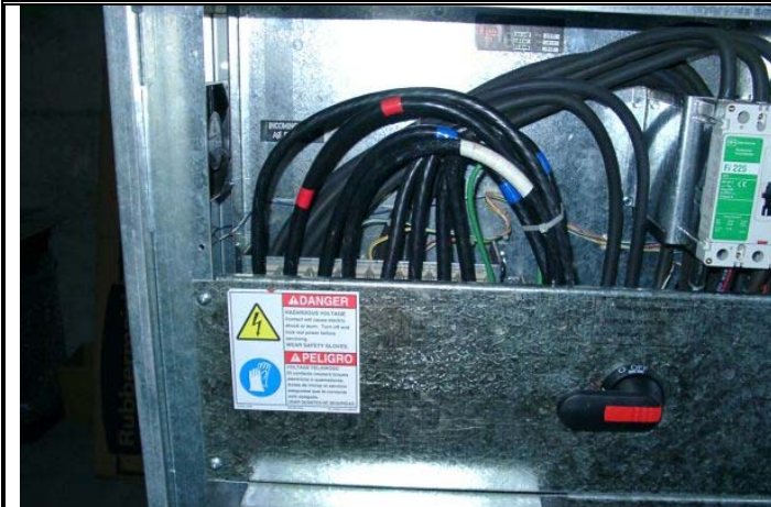
Parking Structure #1 Unit 413
