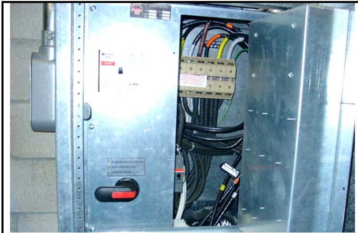
Parking Structure #4 Unit 880
