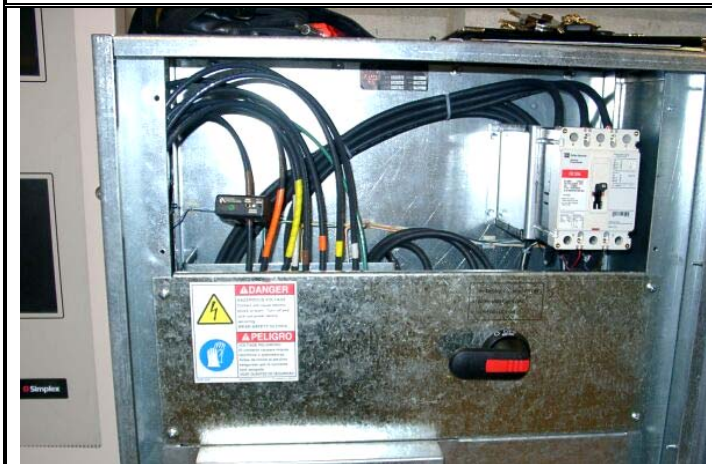
Parking Structure #6 Unit 950
