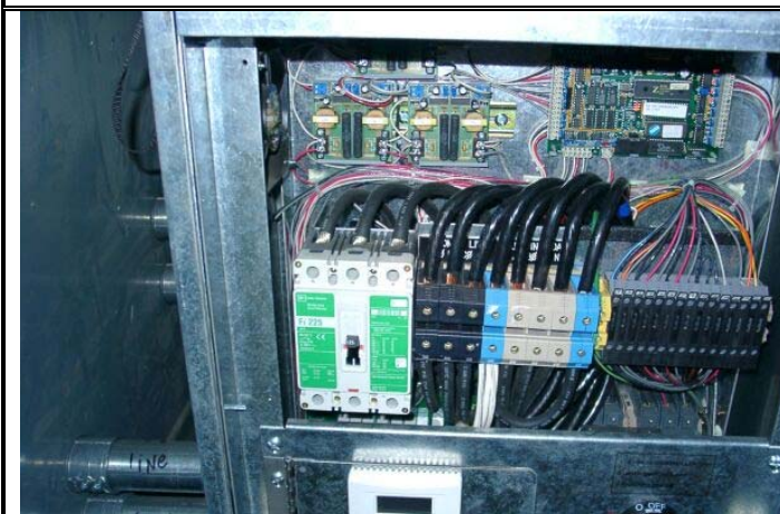
Parking Structure #1 Unit 894
