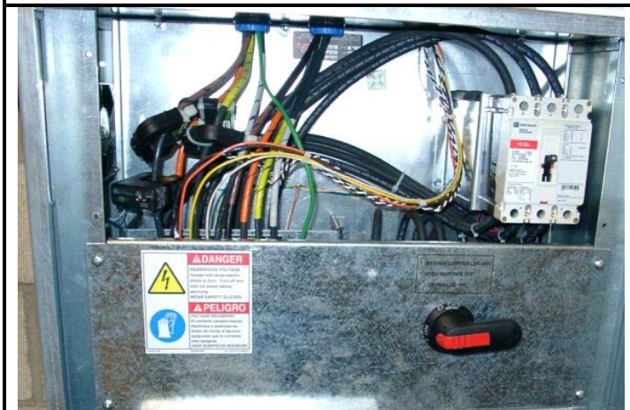
Parking Structure #5 Unit 984
