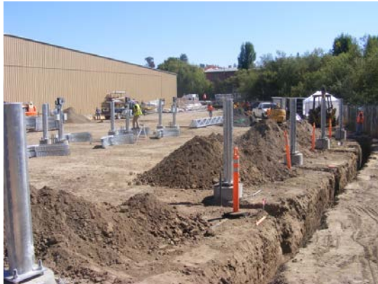
FIGURE 4: SONOMA WINE COMPANY MOUNTING POST INSTALLATION
