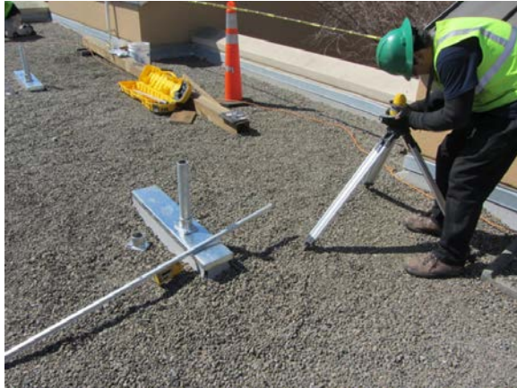
FIGURE 9: ROOF INSTALLED MOUNTING POST
