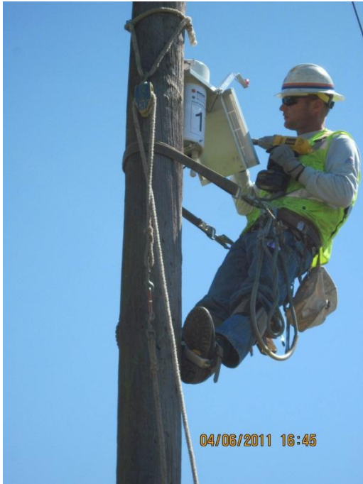
Figure 6-3. SMUD lineman installing one of the secondary stations in Sacramento, California
