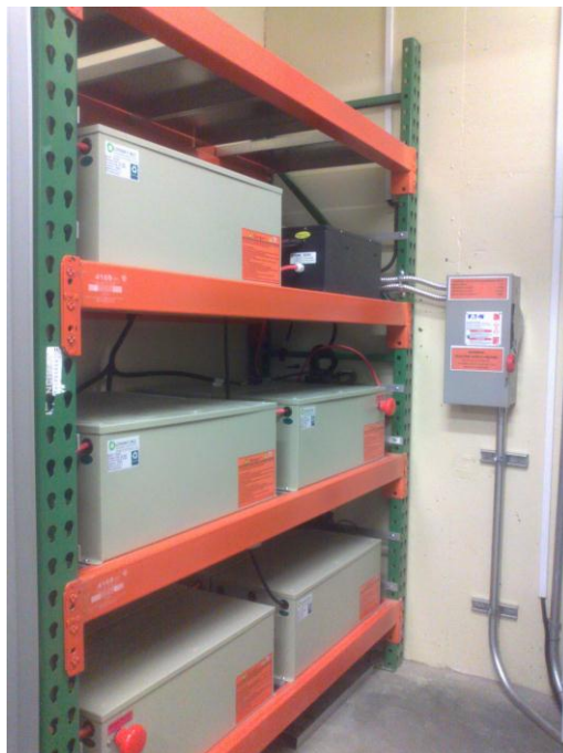
Figure 13: Battery Bank and Battery Management System
