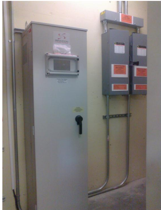
Figure 14: Bi-directional Inverter and Disconnect & Bypass Switches
