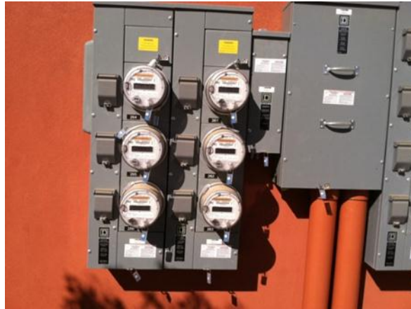
Figure 1: Bank of PG&E Net Meters
