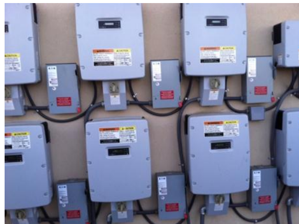
Figure 2: Bank of Individual String Inverters
