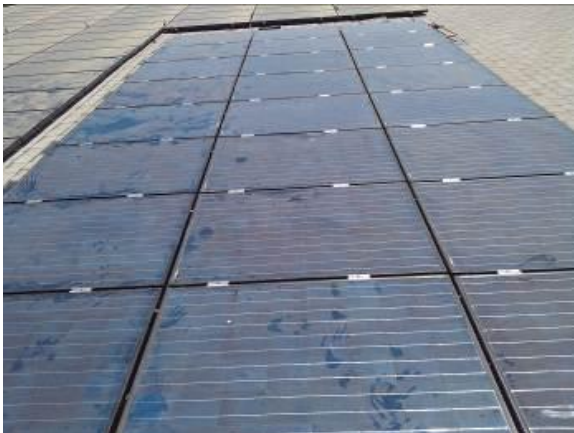
Figure 19: Design schematic and photos of the integrated PVT system installed at West Village.
