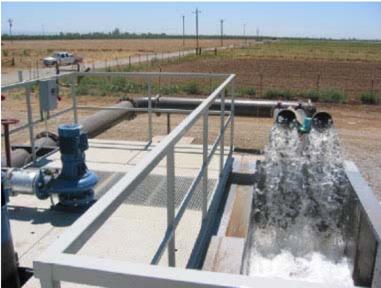
Flow meters located in each pipe.
