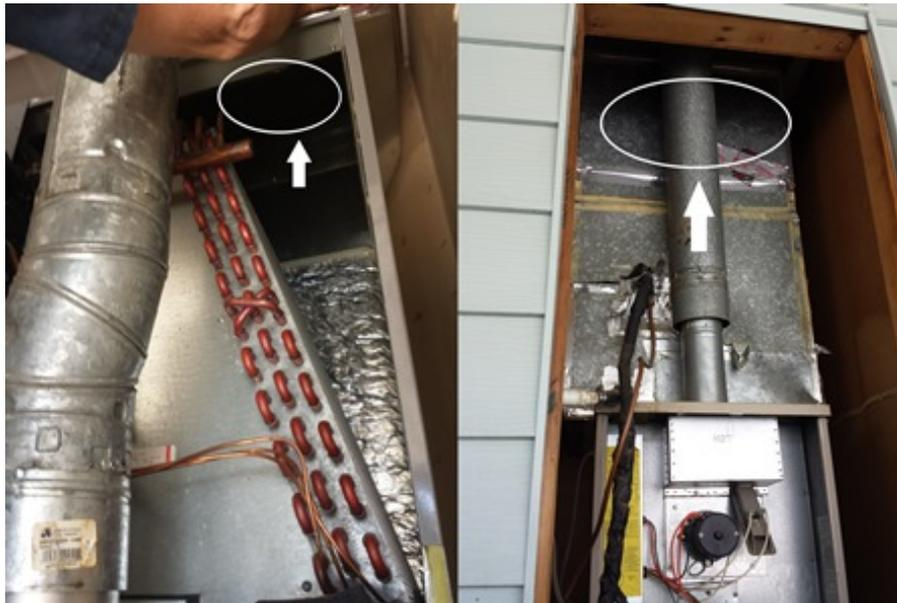
Figure 5.2: Recommended Locations for Supply Air Temperature/humidity Sensor Placement in Upflow Systems
