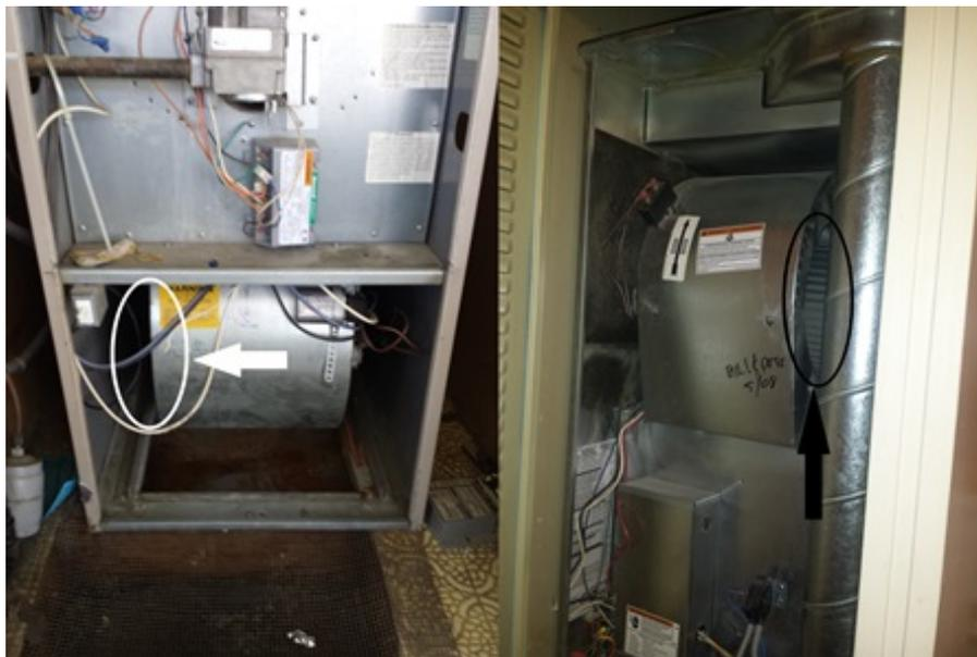
Figure 5.1: Recommended Locations for Return Air Temperature/humidity Sensor Placement
