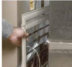
TrueFlow® Plate #14 with 2x20 spacer at filter slot between the return and the air handler.
