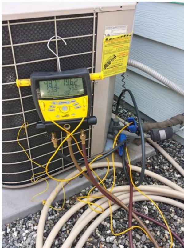
Figure 3.1: Typical Installation of the Digital Manifold Gauge Set
