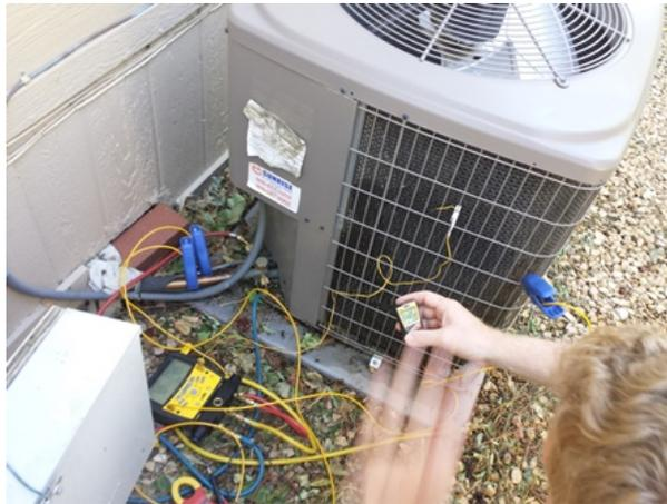
Figure 3.9: Typical Measurement of Outside Air Temperature
