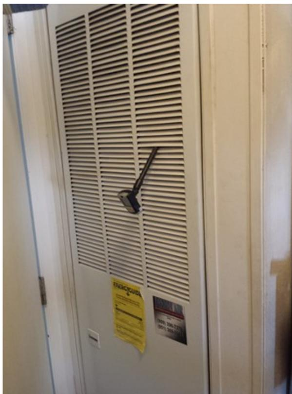
Figure 2.2: Typical Return Air Temperature Measurement
