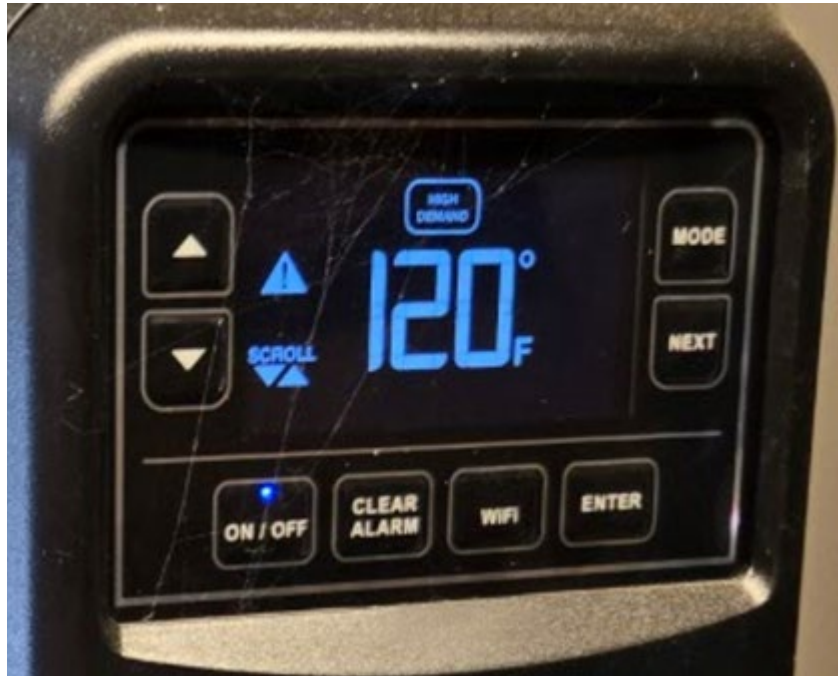
Figure 16. On-Site HPWH Digital Screen
