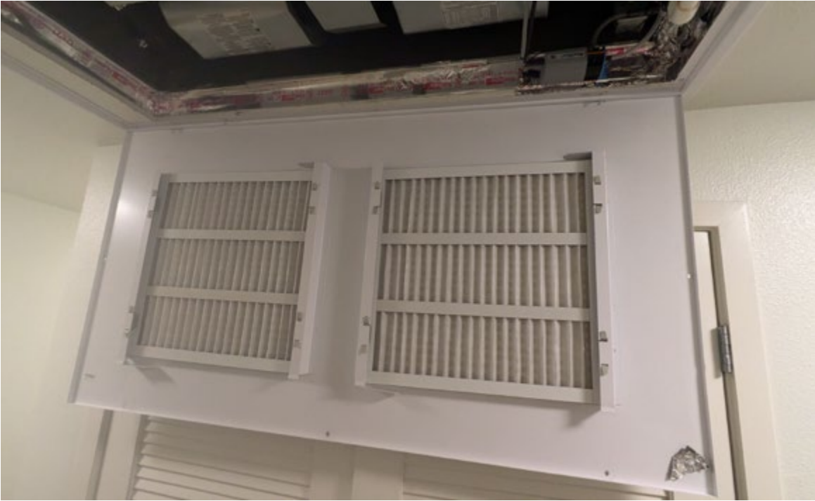
Figure 6. In-Unit HVAC Indoor Forced Air Unit (FAU) with Ceiling Access Cover
