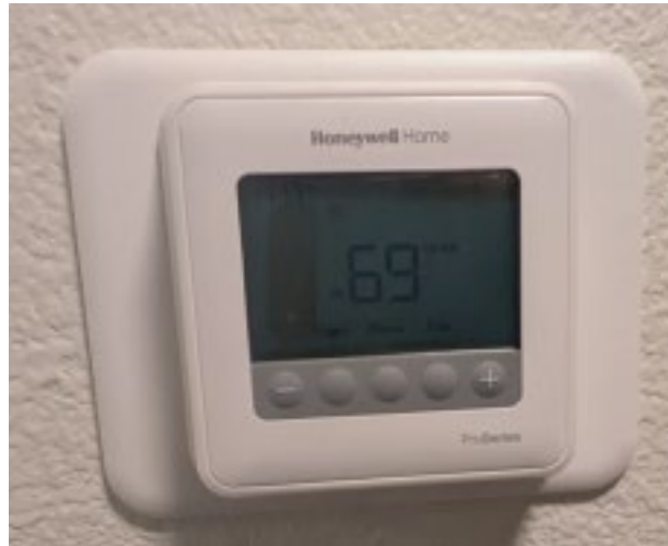
Figure 4. In-Unit HVAC Thermostat Control
