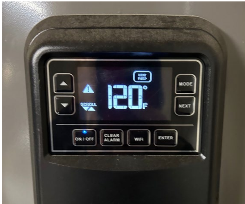
Figure 20. On-Site HPWH Digital Screen
