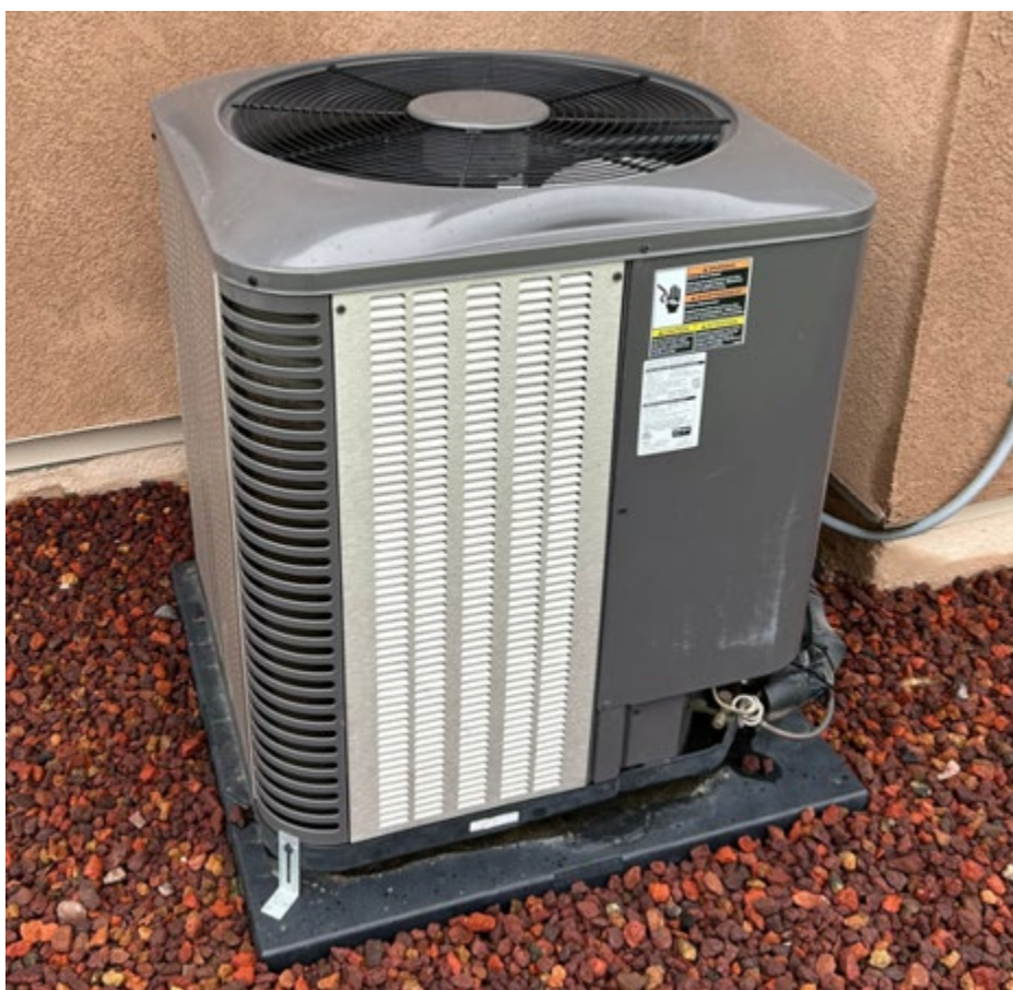
Figure 19. HVAC System Outdoor Condensing Unit
