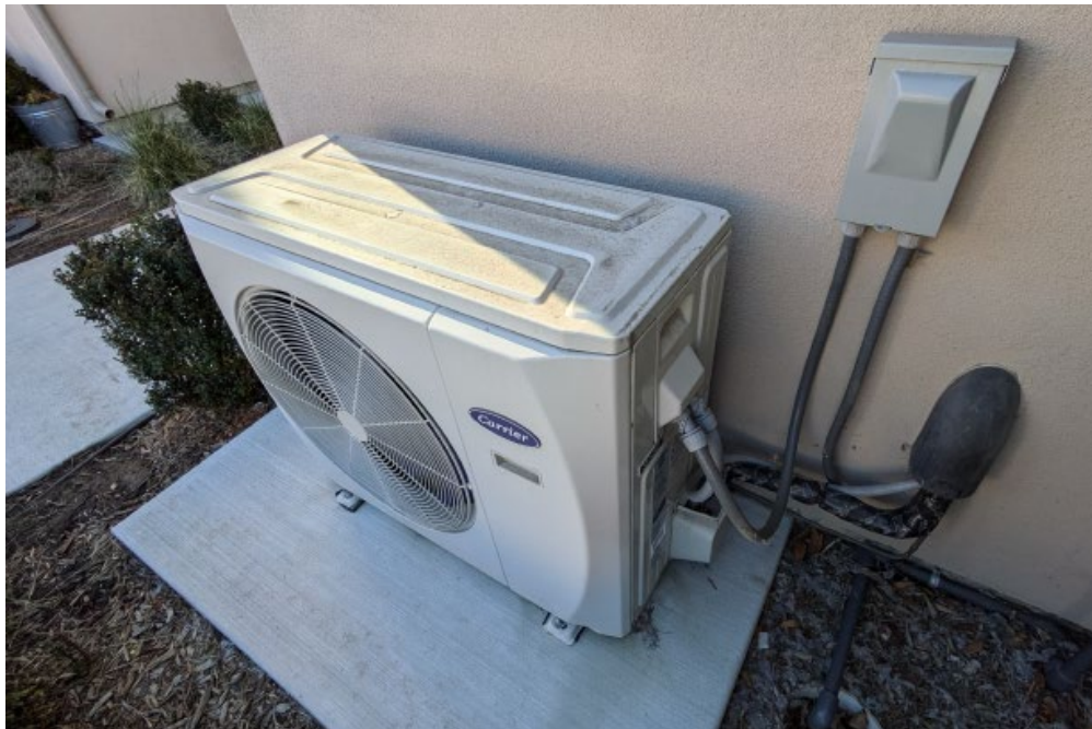
Figure 5. HVAC System Outdoor Condensing Unit
