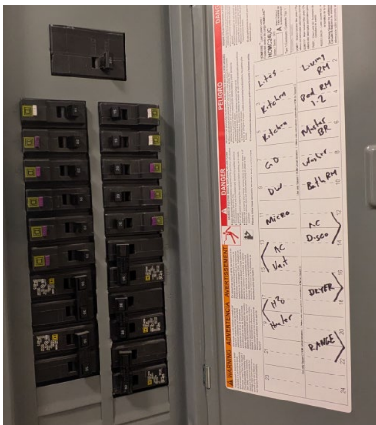
Figure 3. In-Unit Electrical Panel
