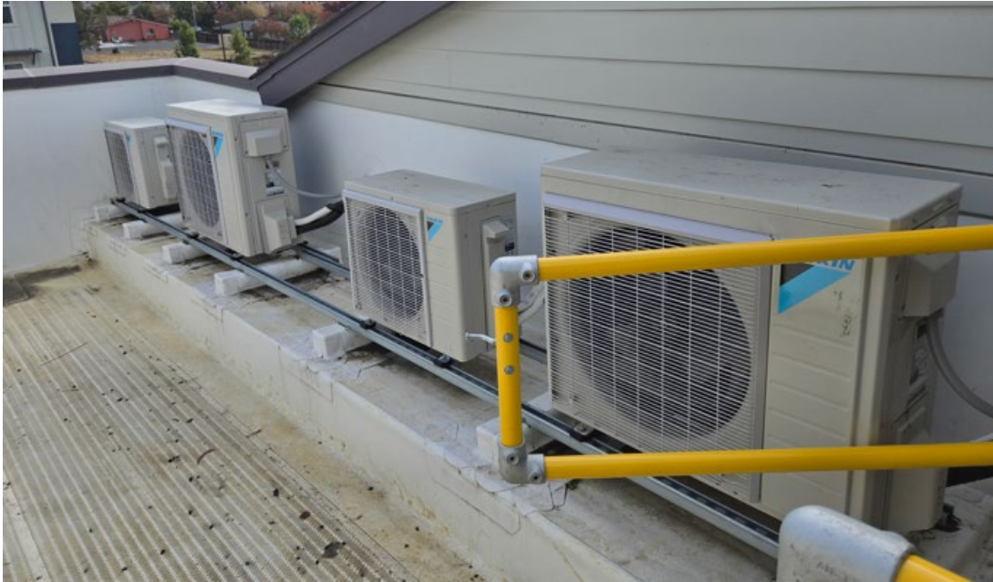
Figure 14. HVAC System Outdoor Condensing Unit
