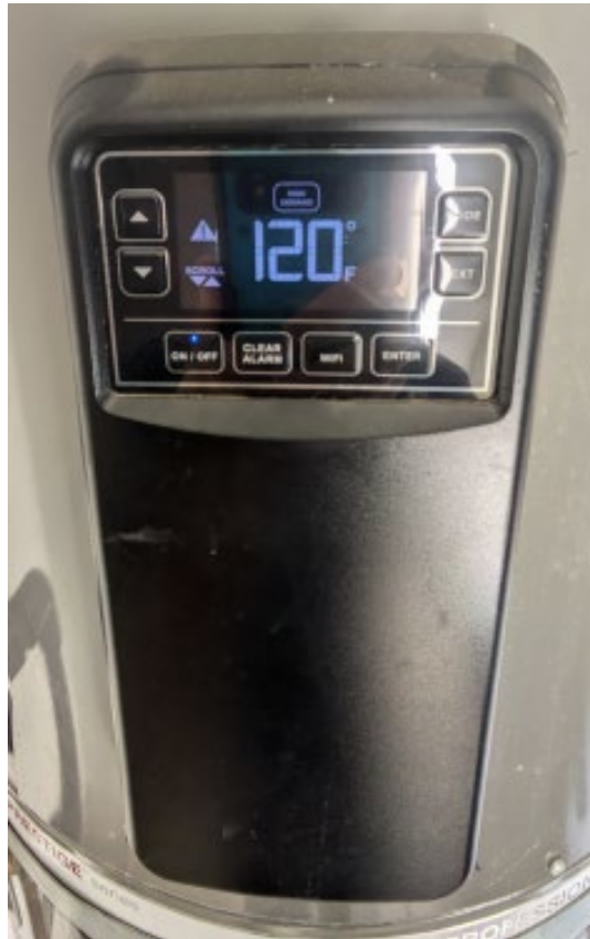
Figure 8. On-site HPWH Digital Screen
