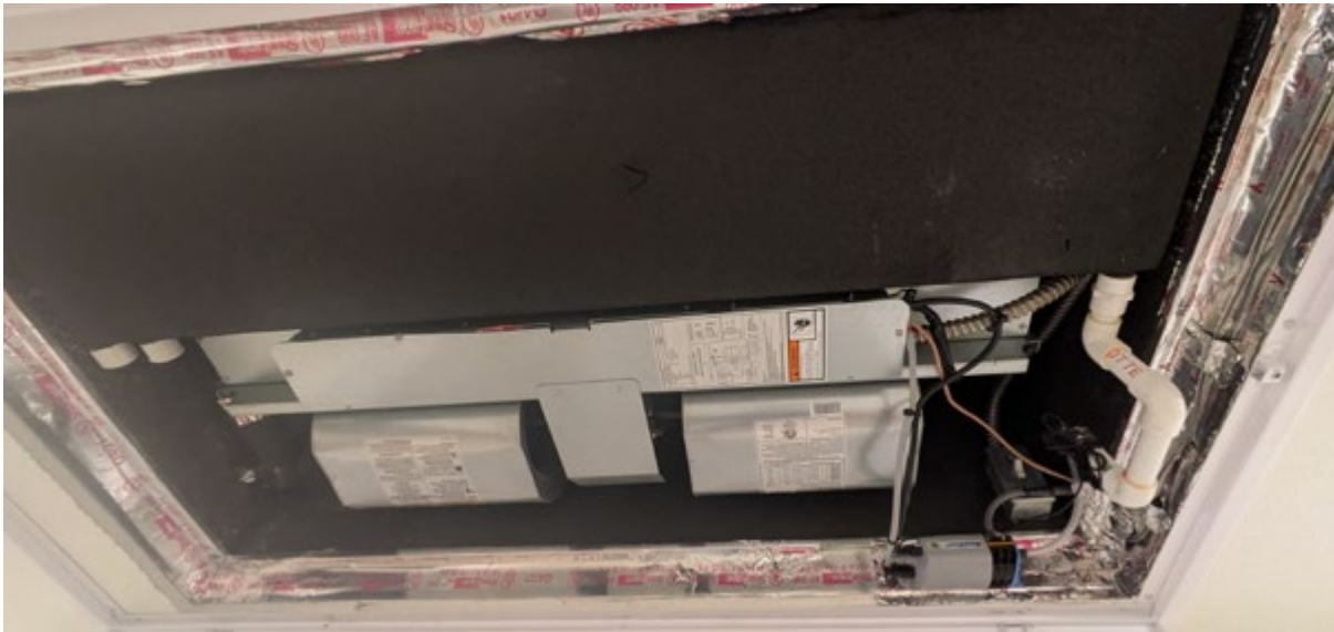
Figure 7. In-Unit HVAC Indoor Forced Air Unit (FAU) Exposed
