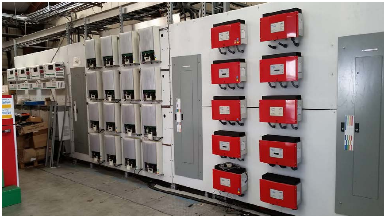
Figure 7 Residential PV inverters installed at PG&E Applied Technology Services Center in San Ramon CA
