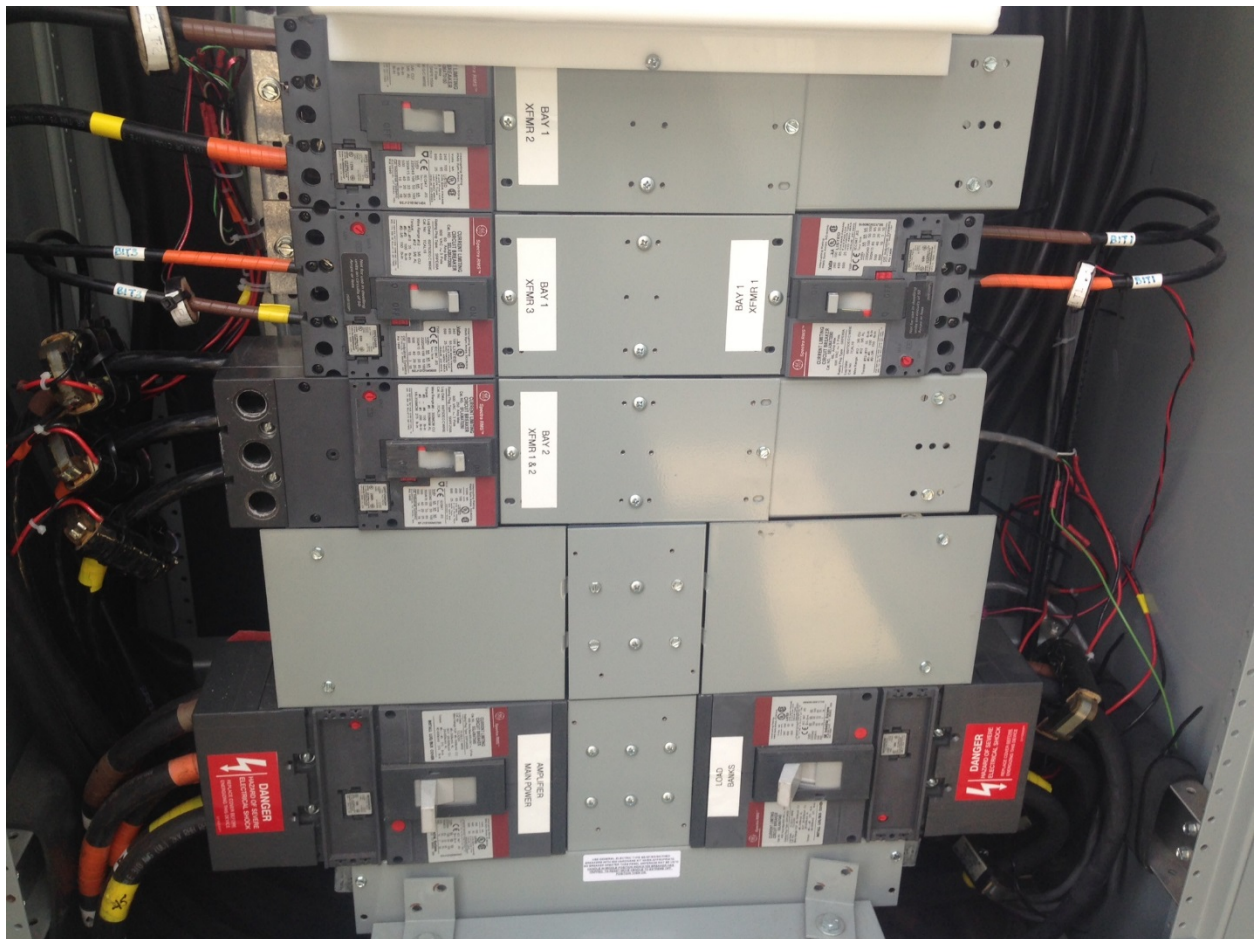
Figure 11 Measurement system: Breaker panel and current transformers
