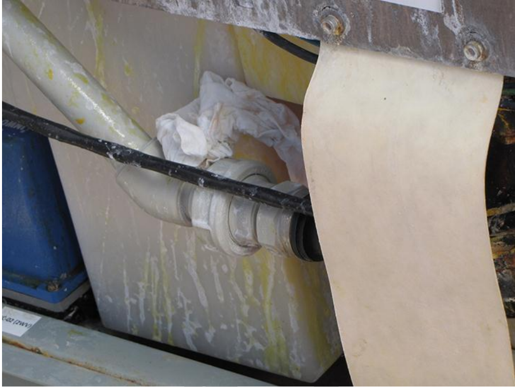
6 - Unit 3 electrolyte residue on electrolyte reservoir
