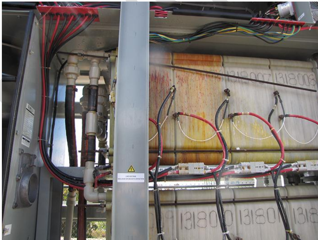
9 - Electrolyte leak location on top left cells of Unit 3
