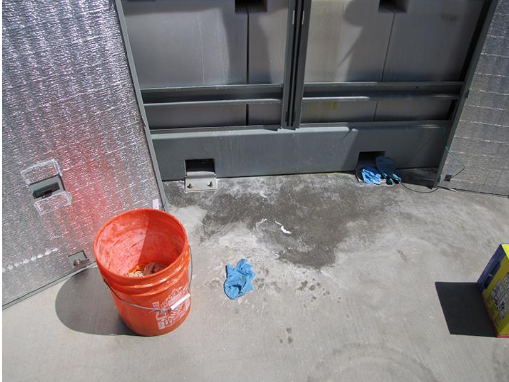
10 - Back side of Unit 3 where electrolyte was spilled outside the cabinets
