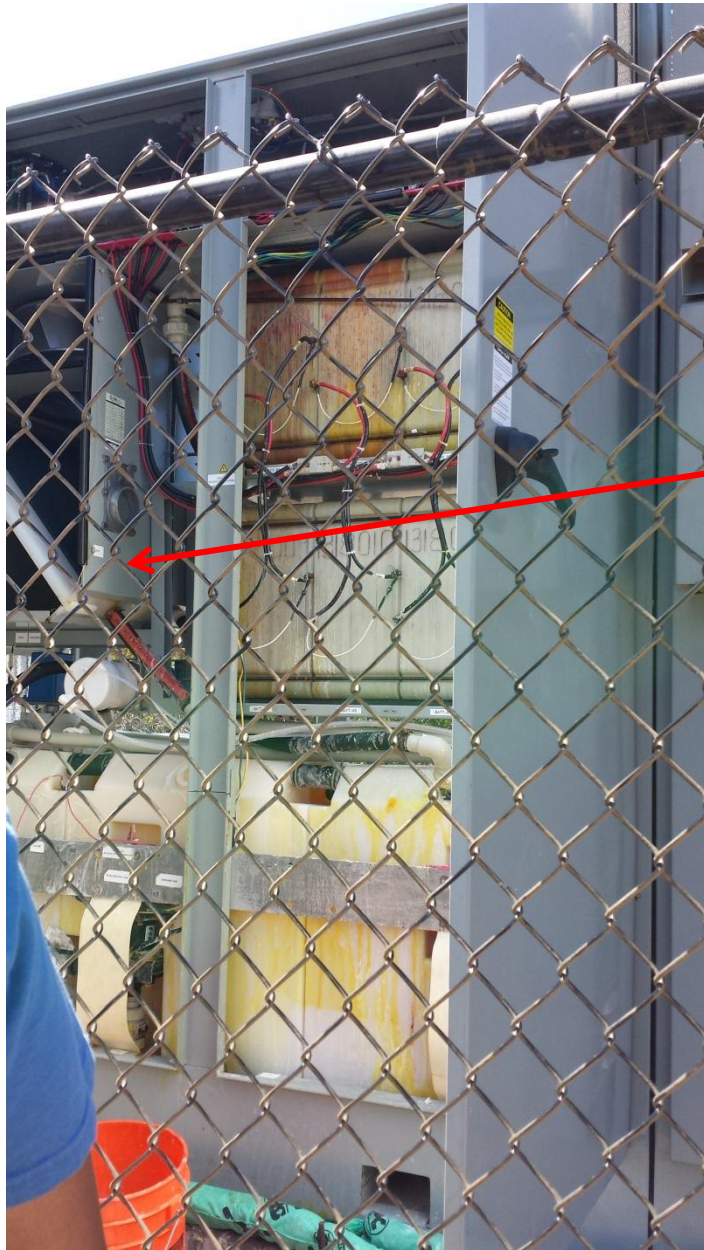
3 - Unit 3 broken threaded rod still within system
