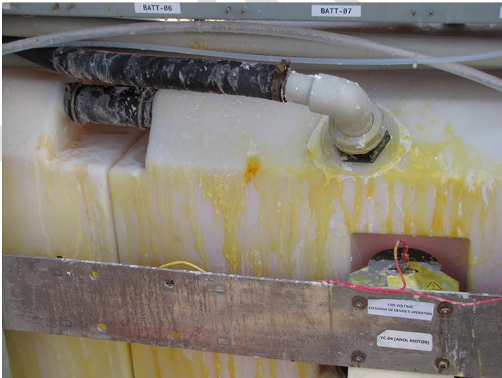
7 - Unit 3 closer look at residue of electrolyte reservoir
