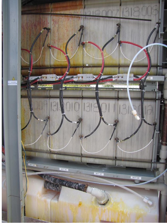
8 - Unit 3 broken threaded rod with residue electrolyte
