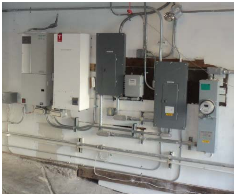
Figure 16 - Residential Li-ion Installation
