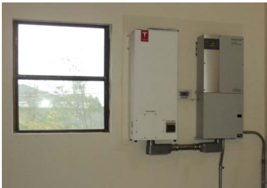
Figure 15 - Residential Li-ion Pilot Installation
