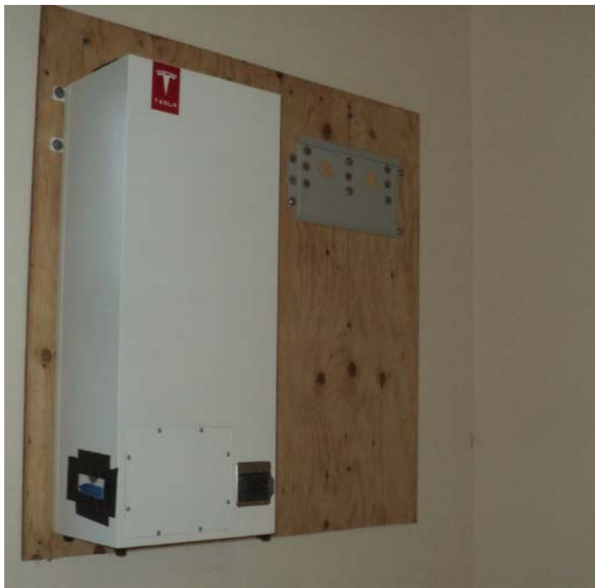
Figure 193 - Mounting the Residential Li-ion System
