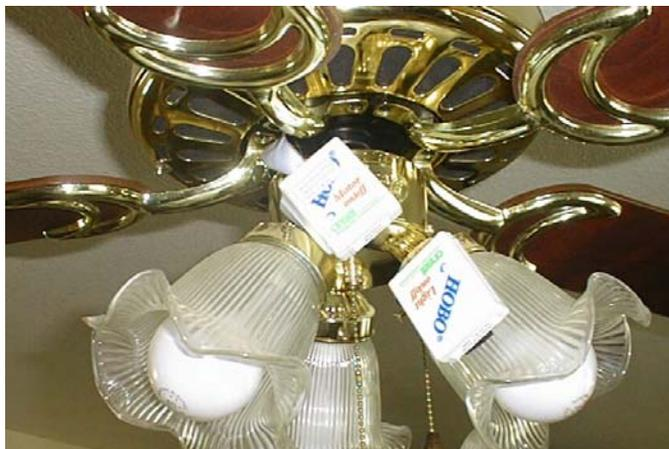
**Figure 15: Data Loggers Mounted with Hook and Loop Fasteners**
