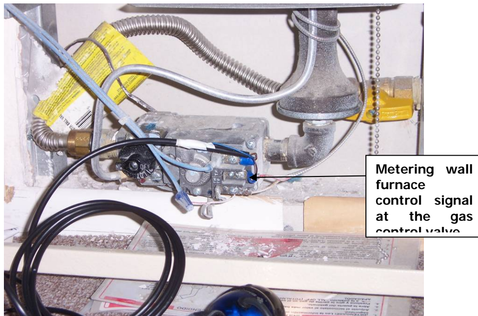
Figure 66: Wall Furnace Installation
