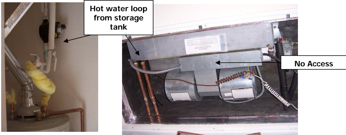
Figure 65: Hydronic Fan Coil Unit
