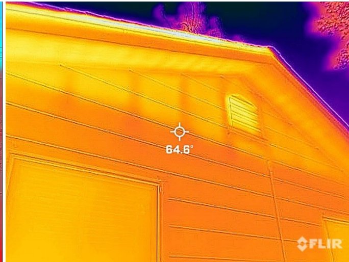
FLIR™ infrared image showing a section of insulated wall
