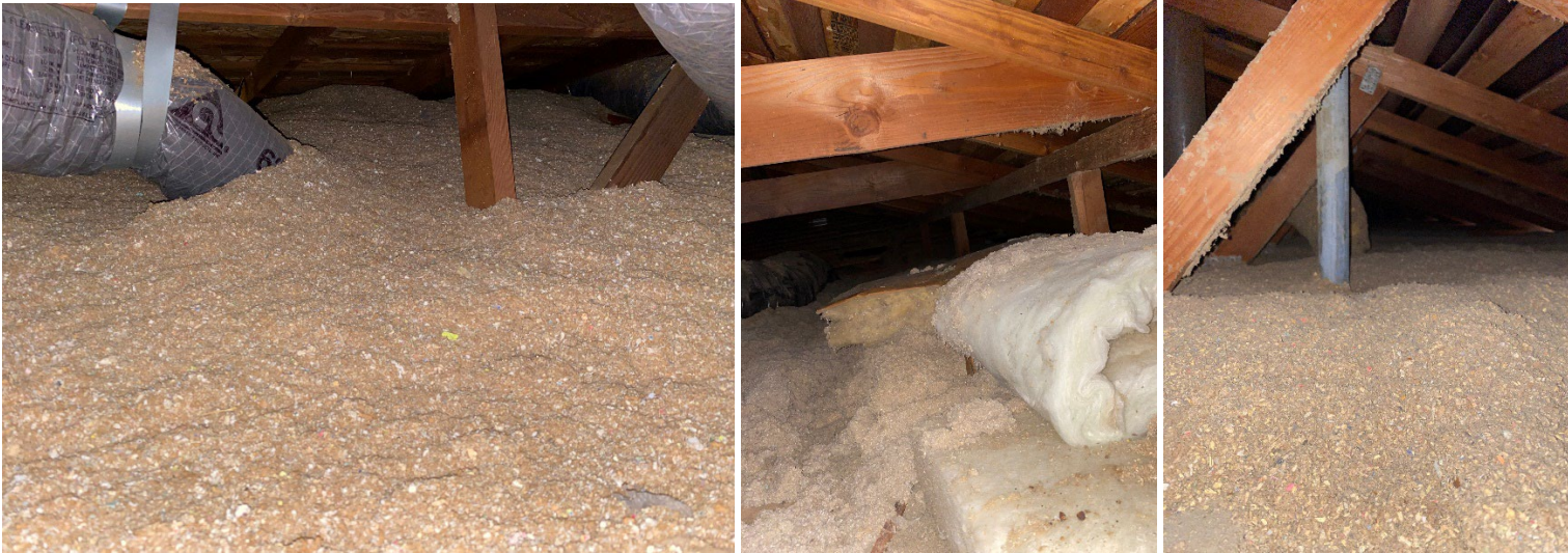
Images showing insulated ceiling/attic.
